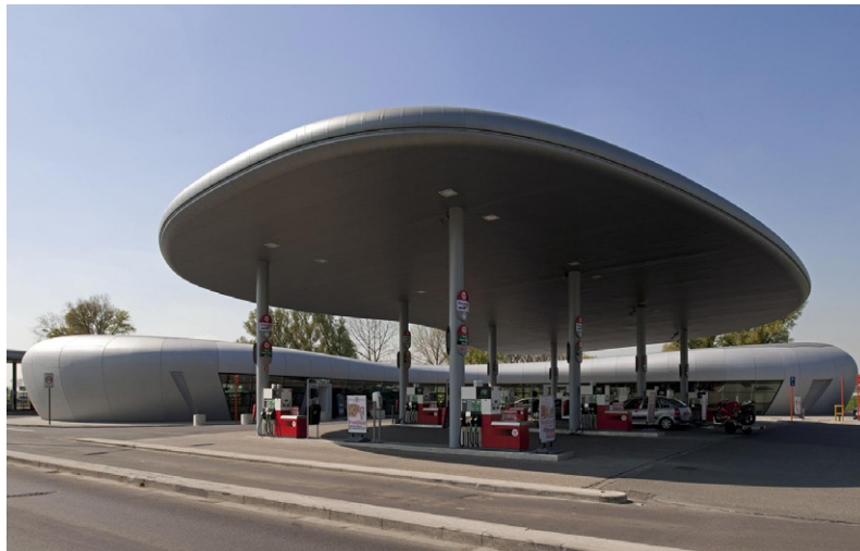
Texaco, Kruibeke (BE) Bontinck architecture and engineering bvba
