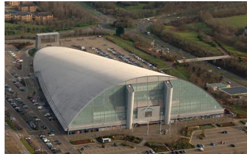
Xscape, Milton Keynes (GB) FaulknerBrowns Architects
